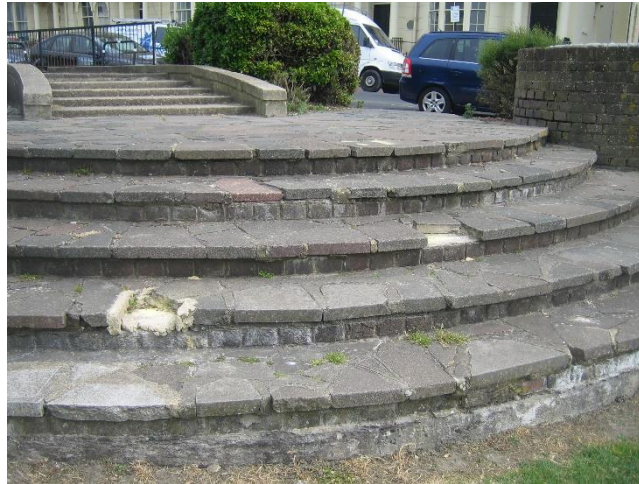
It won't be long until someone falls down these steps with their missing edges
