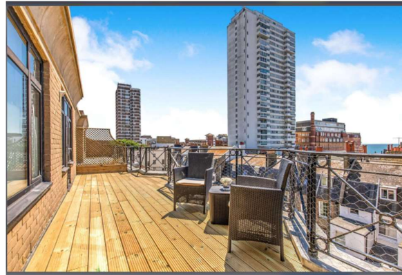
Estate Agent Photograph of the fourth floor terrace of Russell House – chicken wire instead of required 1.5m high obscured glass!
