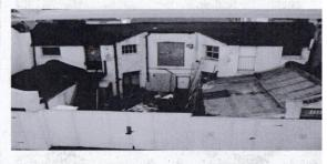
Although the building is in very poor condition the basic structure is almost intact and you can easily pick out the Hay Loft (centre First Floor), the Stables Lads' accommodation to left and right of the Hay Loft (accessible only by ladder) and the pedimented carriage entrances to the right and left of the courtyard.
