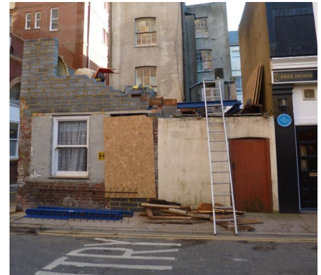
Work in progress on 122 Kings Road
